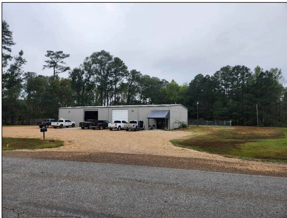
Figure 14. Resource No. C-2, facing southwest.
