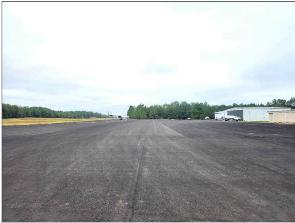
Figure 12. Resource No. C-1, facing north.
