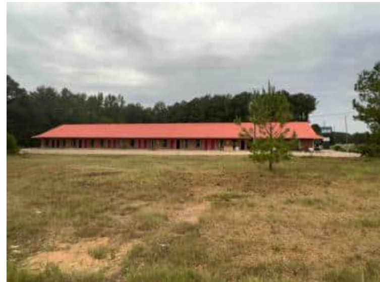
Photo 4 View of west adjacent Economy Inn, facing west from the site.
