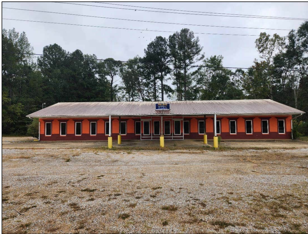
Figure 15. Resource No. C-3, facing southeast.
