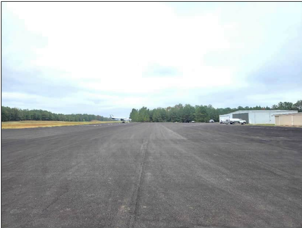
Figure 14. Resource No. C-1, facing north.
